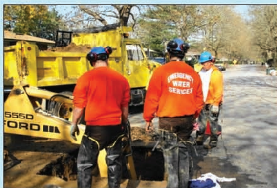
SHWD crew performs repairs on distribution system.
