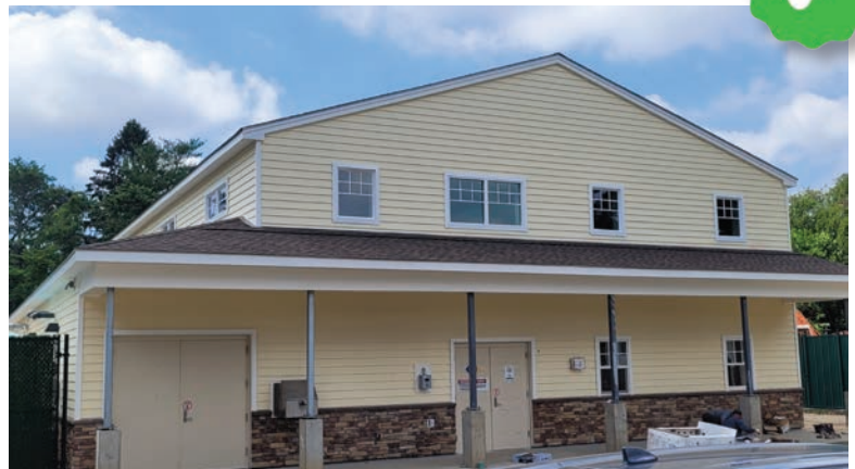
Plant No. 8 recently returned to service with new AOP and GAC treatment systems.
