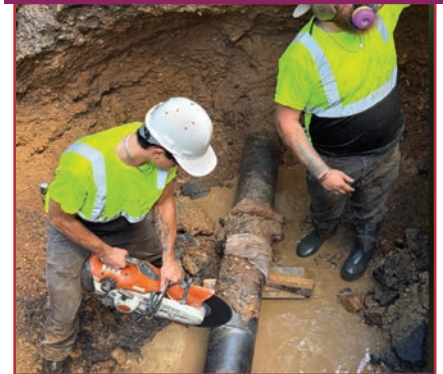
SHWD maintenance mechanics seize the opportunity of a water main leak on W. Rogues Path to install a new 8" valve. The new valve will improve efficiency of shutdowns with any future issues.
