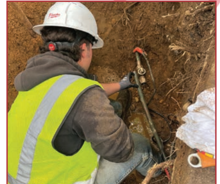
SHWD maintenance mechanics seize the opportunity of a water main leak on W. Rogues Path to install a new 8" valve. The new valve will improve efficiency of shutdowns with any future issues.
